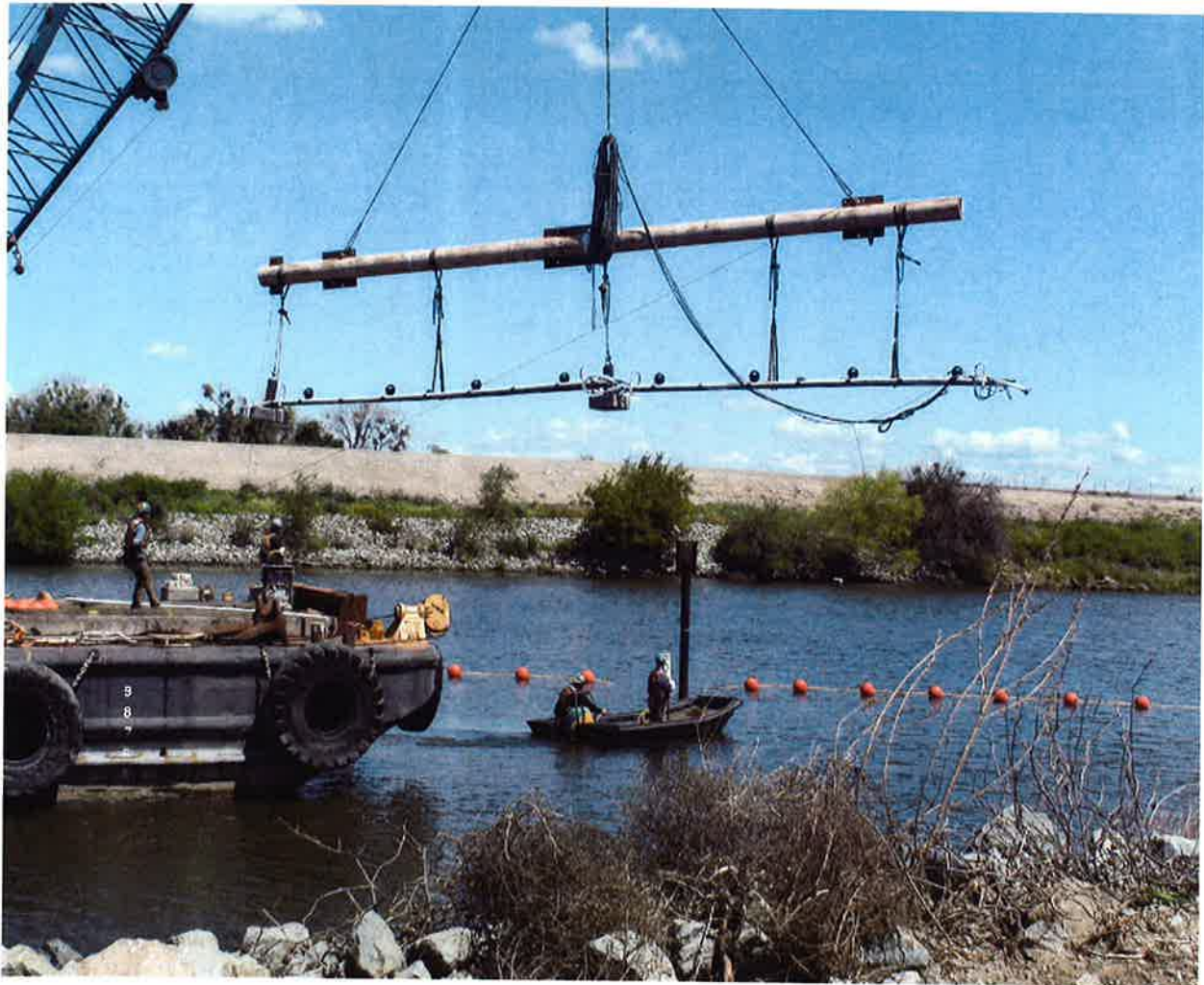
Figure 8. Close-up of NPB assembled modular frames being installed
