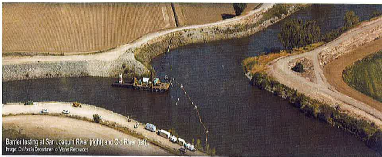
Figure 5. Aerial of Non-Physical Barrier (NPB) installation
