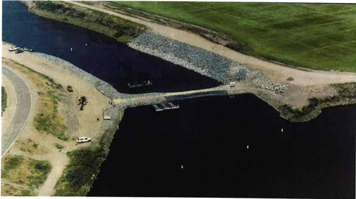
Figure 3. Aerial of spring Head of Old River temporary rock barrier
